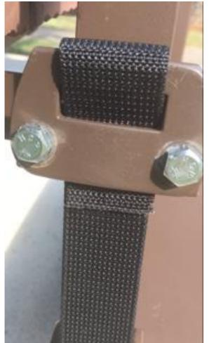
Hang the platform, the straps are pressure fit with the aluminum pins.
