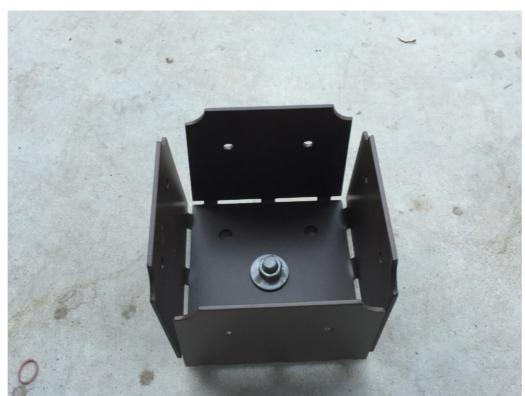
Galvanized plate goes UNDER the boot That keeps things from moisture buildup
