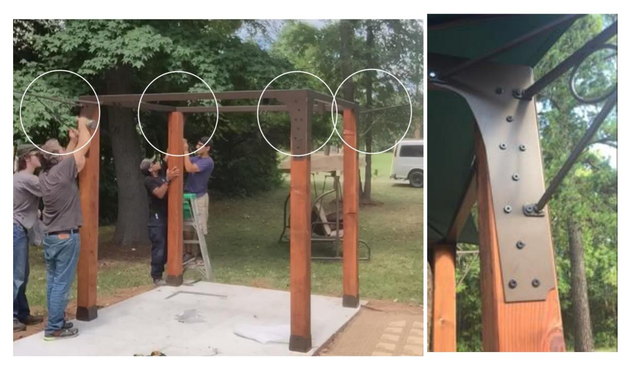
Check posts for level, then mount the canopy arms, using two of the headlock holes, and one hole that uses a small 1/4" nut and bolt.
