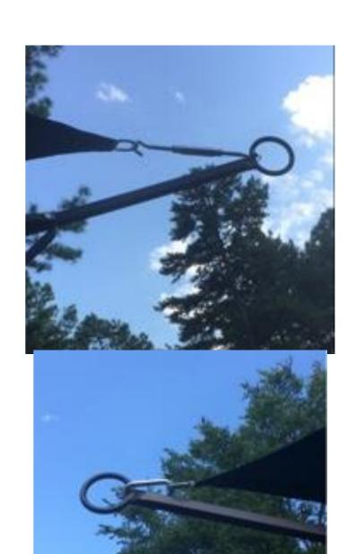
Hook the canopy up, keep the turnbuckles extended and don't tighten them until you place the PVC pipe on the studs.
