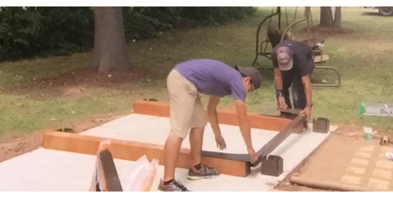
Layout two posts and attach the 'short' crossbar, The sides of the crossbar flanges should sit about 1/4" from the outside edge of the wood.
