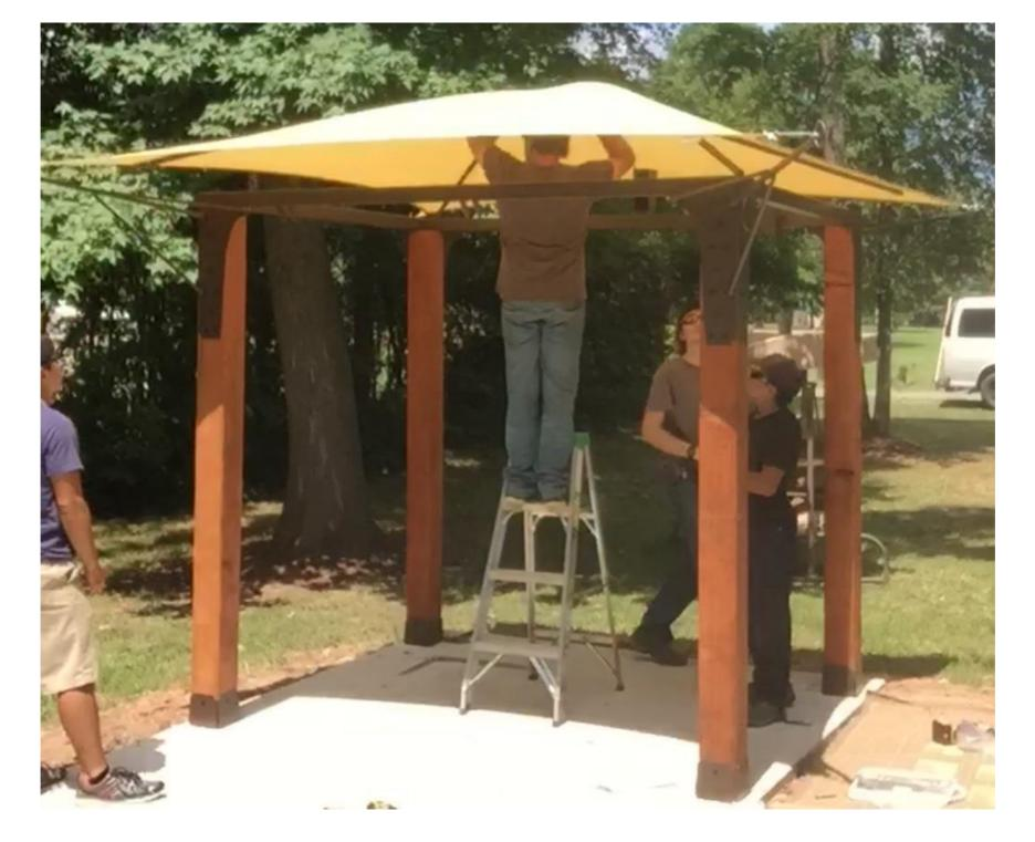
Put PVC tubes in center cross fitting, stretch the canopy upwards, and have another person insert outside ends over the studs that are welded onto canopy arms.
