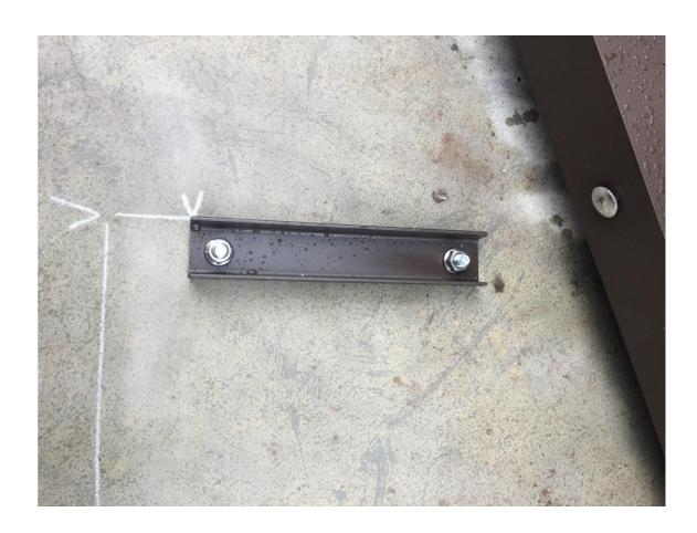
After you move the platform out of the way Mount the brake stop 2" in from edge of where platform will be as shown in picture with the 3/8 anchor pins.
